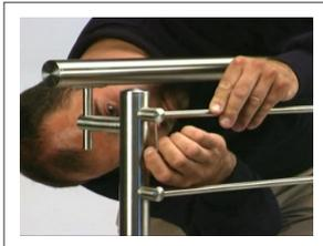
Secure with grub screw using hex head key.
