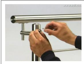
Fix to the post with M6 countersunk screw.
